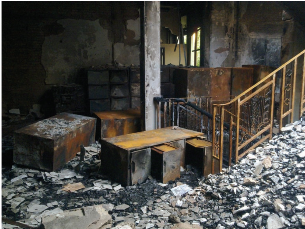
Rubble and burned-out filing cabinets on second floor of the central staircase of the old wing of the Khon Kaen provincial hall, which was set afire by protesters on May 19, 2010. © 2010 Human Rights Watch
